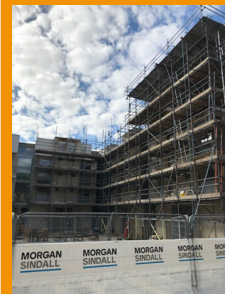
Courtyard access scaffolding
