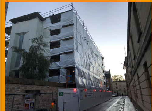
Courtyard access scaffolding
