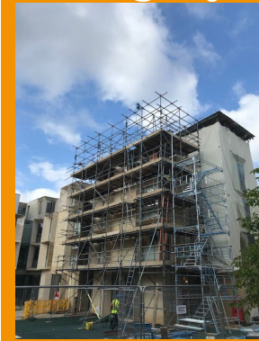
Courtyard access scaffolding
